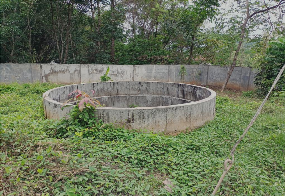
Figure 28: Open well in the campus
